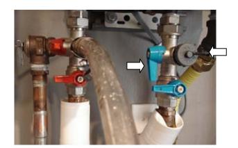
17. Put the hot water drain hose back into the bucket and open the cold water main valve. This procedure will flush out the heater with fresh cold water. Flush for at least 5 minutes or until 20 gallons of water has passed through the heater
