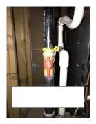
**ELECTRIC FURNACES**: heat will turn off with a clogged condensate drain (the white pipe besides the furnace). Snake out any obstruction to the drain and clean yearly with pouring bleach down the line.
